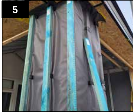
Begin to place 2 x 25x50mm battens above the corner post and fix back using the winged screw. Maintain 12mm offset to top clip as with the rest of the battens (excluding flat roof).
