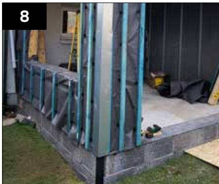
Completed structural corner post shown, at this point the CSB can be fitted to the build.
