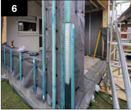
Fit 2 x 25x50mm battens on either side of the corner post using the winged screw.
