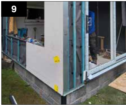
Calcium silicate board starter profile and the calcium silicate board are fitted over the structural corner post as shown.
