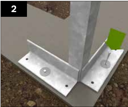
Drill 10mm holes in the concrete footing centrally through the two large holes in SLP002 structural post. Temporarily clamp the post in place using SLP004 kit (M8 anchor bolts, washers and packers). Note: hup! build hidden in image for clarity.
