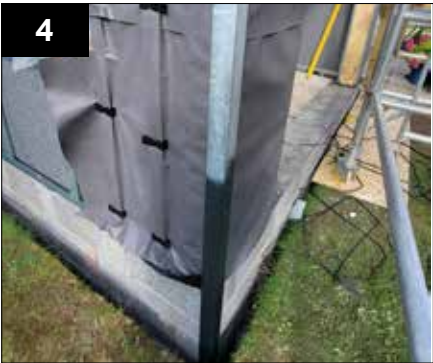
Secure the structural post into the hup! corner using GPHS fixings through the pre-drilled holes.
