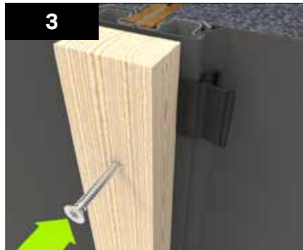
Position a 25mm batten, treated timber (optionally provided) or alternative, against the clips trapping the membrane in place. At apertures this batten is positioned inline with the opening. Secure the batten to the walling full and half clips using the winged fixing screw (provided with battens). Please Note : - Excluding flatroof, the battens will be shorter than the clip length and should be set down from the eaves level or other air flow obstructing roof elements by 12mm to allow for ventilation.
