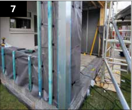
After fitting the battens the L shaped steel profile can be fitted to the battens. Use GPHS fixings at 300mm centres.
